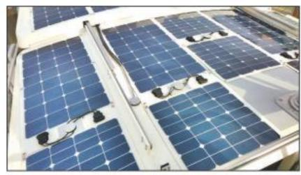
This array of semi-flexible solar panels on a motoryacht employs SunPower cells (note the absence of fingers or busbars on the top of the cells). All the panels have 32 cells of the same size, but due to space limitations the cells have been cut in half on some panels. For a given level of sunlight, all the panels will reach a similar voltage, but the ones with half-sized cells will deliver half the amperage.
